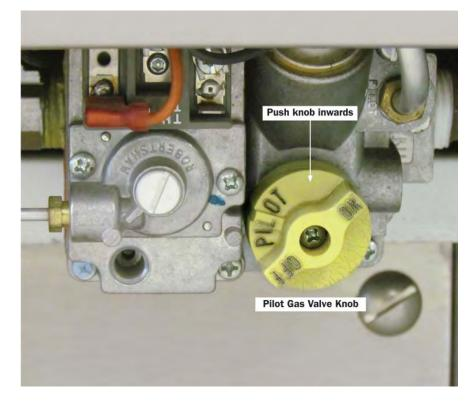
Push in and hold the pilot gas valve knob, and while holding, push the red spark ignition button to light the pilot. (When griddle is first installed, it may take longer than 90 seconds to bleed the air from the gas line).
